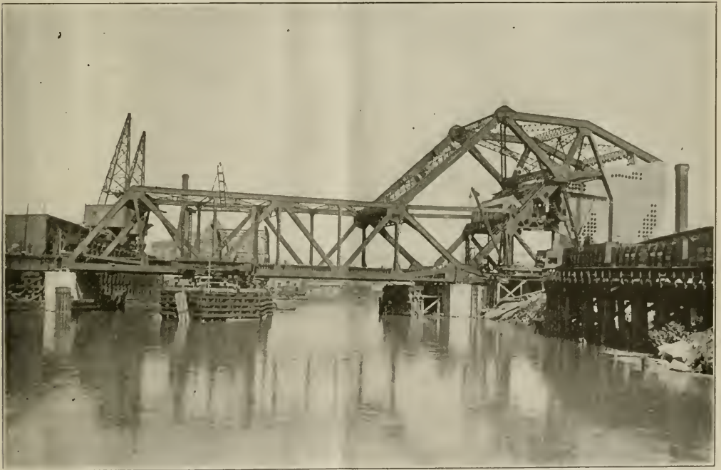
CHICAGO & NORTH WESTERN RAILWAY BASCULE BRIDGE OVER THE CHICAGO RIVER NEAR DEERING, ILL. VIEW SHOWS BASCULE BRIDGE IN POSITION, READY FOR TRAFFIC.
